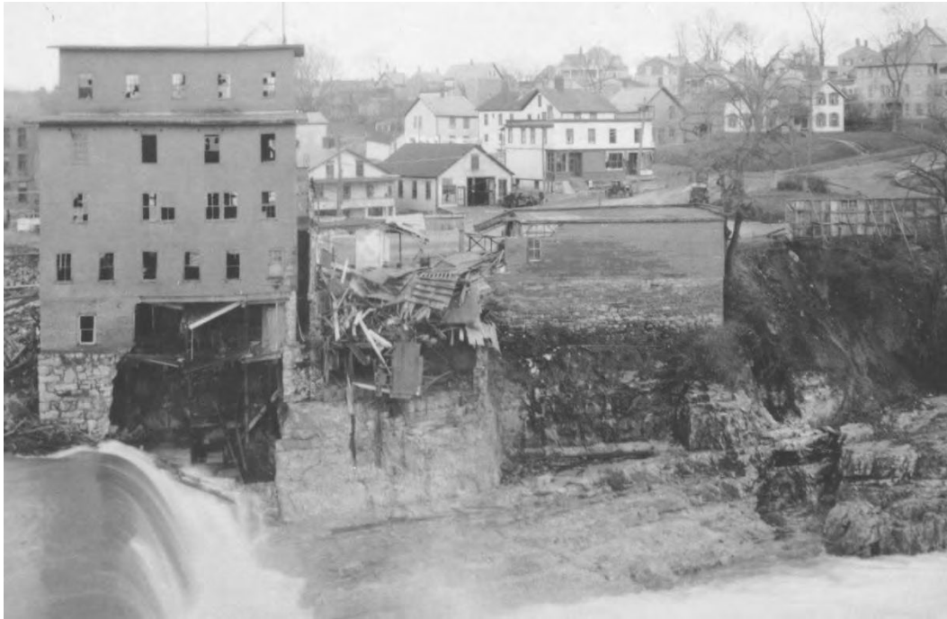
Figure 49. Detail of a view looking from the Colchester / Winooski side of the Winooski River towards the old grist/flouring mill on the Burlington side at the dam, showing the damage caused by the flood and the dynamite charges (Lois L. McAllister Photographs Collection, Box A19, Folder 10, Item 01, Silver Special Collections, Billings Library Annex, University of Vermont, Burlington, Vermont).
