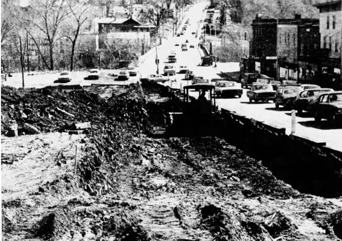
Figure 39. View of the beginning of Winooski's Urban Renewal project on Main Street ( Burlington Free Press April 18, 1974). The bulldozer is operating about where the Brunswick Hotel was located.
