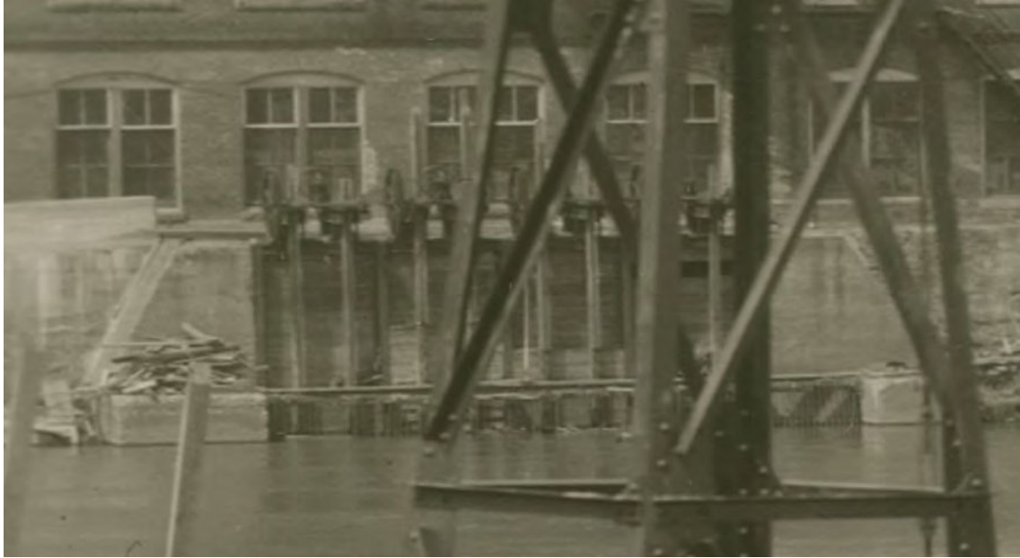
Figure 23. Detail of a 1927-1928 bridge construction photograph showing the head gate control structure for the woolen mills (Lois L. McAllister Photographs Collection, Box A19, Folder 13, Item 02, Silver Special Collections, Billings Library Annex, University of Vermont, Burlington, Vermont).
