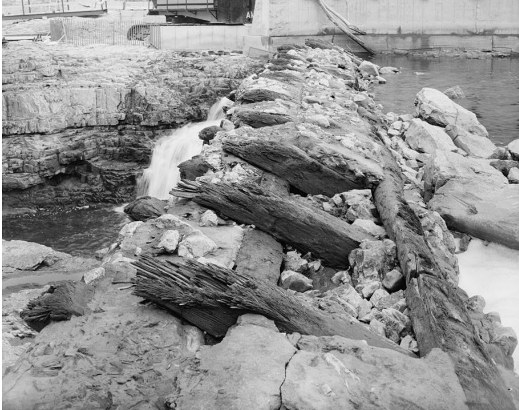
Figure 46. Historic American Engineering Record Documentation, Burlington Woolen Mill Company Dam, VT-23-A-7; Detail of Cribwork, Midpoint Along Top, View West” (photo credit Wayne Fleming 1992; Accessed at: https://www.loc.gov/item/vt0117/ ).
