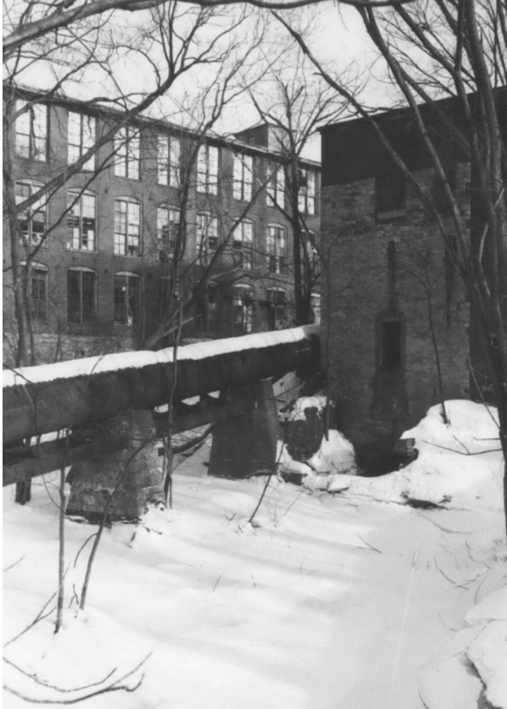
Figure 18. View of the ca. 1880s wheelhouse and penstock leading to the earlier wheelhouse, looking northeast (VT-CH-1298)(Winooski Falls Mill District National Register Documentation, Photograph #7; Credit: Hugh A. Boyd, April 1978).
