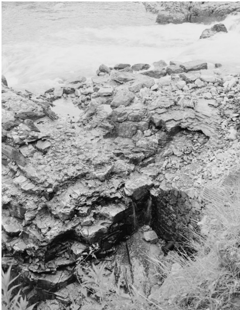
Figure 62. Historic American Engineering Record documentation, Burlington Woolen Mill Company Dam, VT-23-A-9 Remnant of Flour Mill Foundation, East End of Dam, View Northwest (photo credit Wayne Fleming 1992; Accessed at: https://www.loc.gov/item/vt01117/ ).
