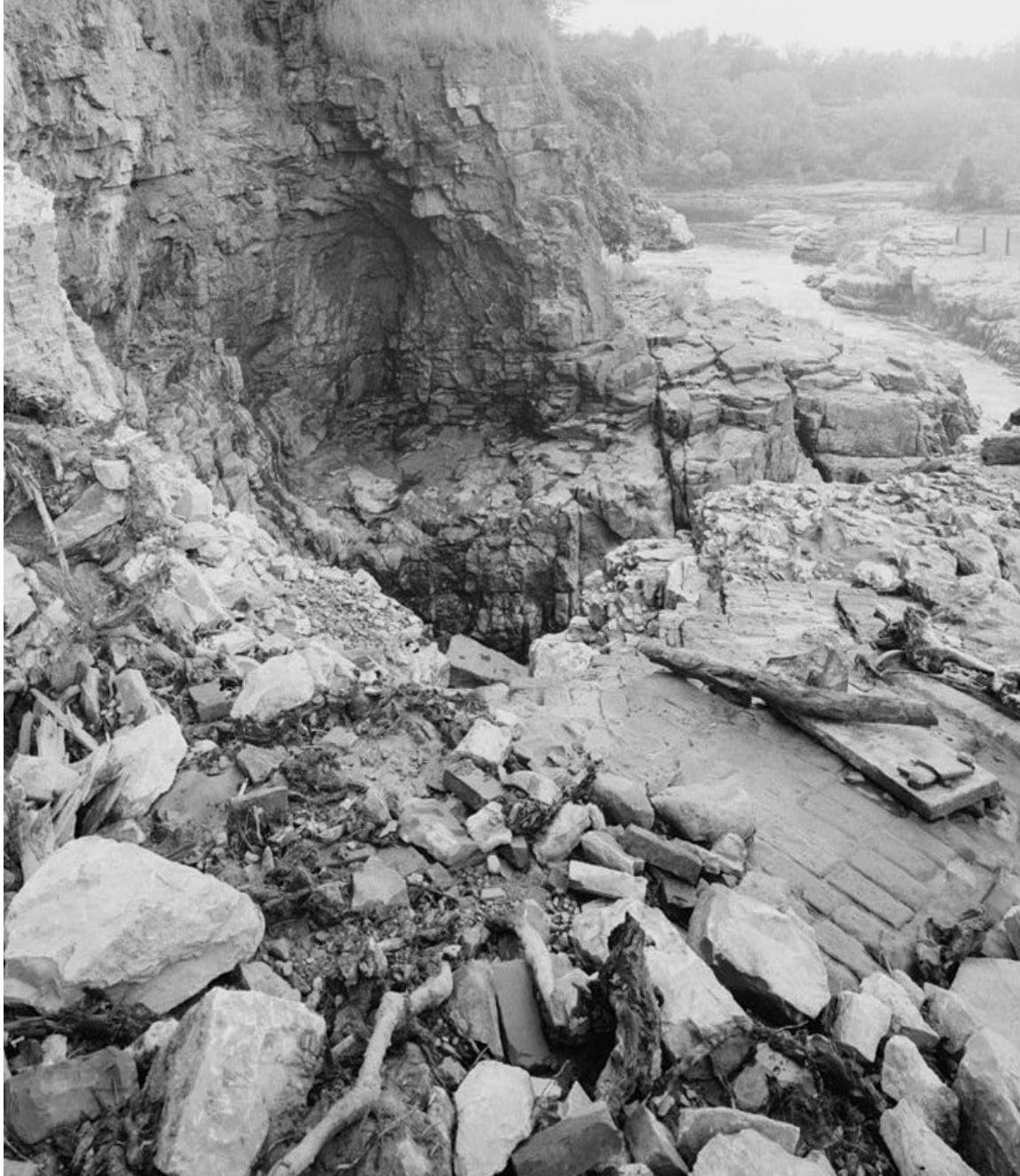
Figure 63. Historic American Engineering Record documentation, Burlington Woolen Mill Company Dam, VT-23-A-10 Remnant of Brick Floor, Flour Mill Foundation, East End of Dam, View Southwest (photo credit Wayne Fleming 1992; Accessed at: https://www.loc.gov/item/vt0117/ ).
