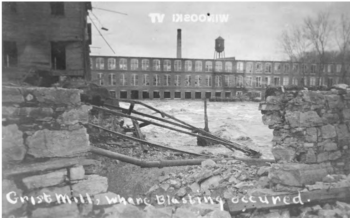
Figure 51. View of the effects of basting near the north side of the mill and the bridge approach, November 5, 1927, looking westwards towards the Colchester / Winooski side of the river (Postcard Collection, University of Vermont Special Collections, Billings Library Annex, Burlington, Vermont).
