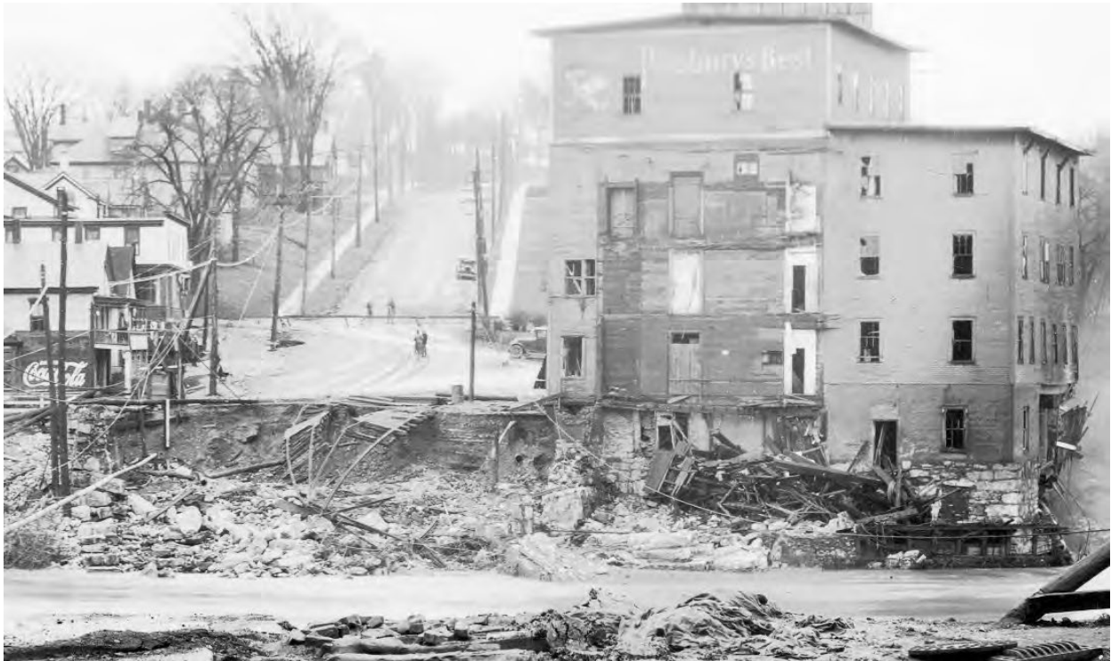
Figure 53. View of the mill building after the flood of 1927, looking south from the Colchester / Winooski side of the river (Lois L. McAllister Photographs Collection, Box A19 Folder 09, Item 04, Silver Special Collections, Billings Library Annex, University of Vermont, Burlington, Vermont).
