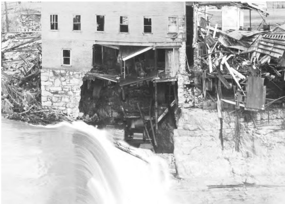
Figure 50. Detail of the previous figure showing the internal structure of the mill and wheel pit (Lois L. McAllister Photographs Collection, Box A19, Folder 10, Item 01, Silver Special Collections, Billings Library Annex, University of Vermont, Burlington, Vermont).
