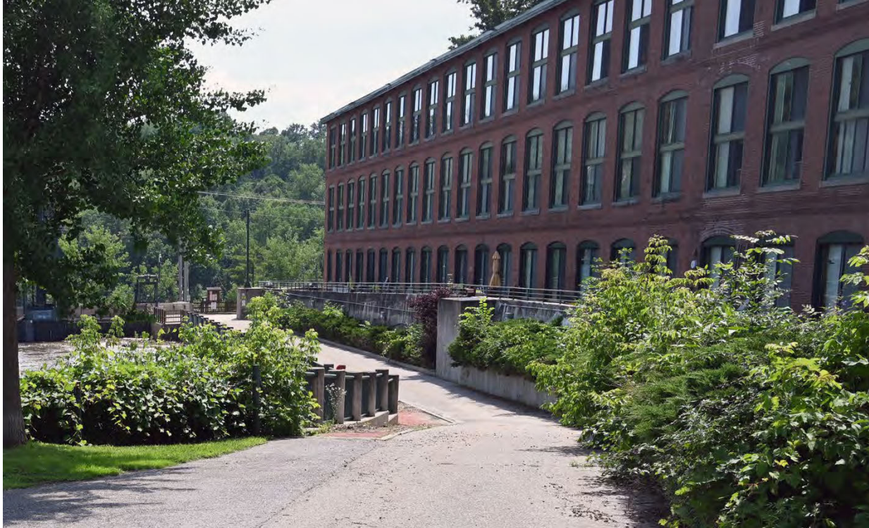
Figure 25. Modern view of the head gate location, now sealed, looking southwards. The gates were located near the point between the two halves of the building meet.
