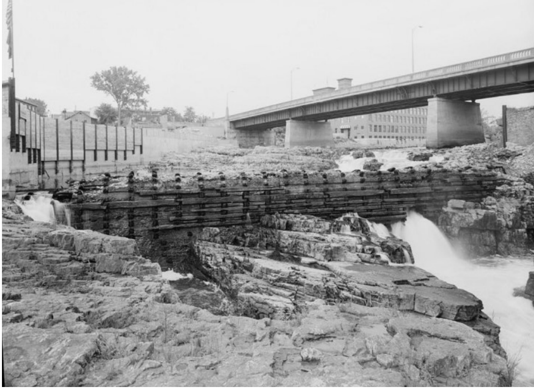
Figure 44. Historic American Engineering Record Documentation, Burlington Woolen Mill Company Dam, VT-23-A-2; View Northeast From the West Bank, Routes 2 & 7 Bridge and Champlain Mill (HAER No VT-11) In Background” (photo credit Wayne Fleming 1992; Accessed at: https://www.loc.gov/item/vt0117/ ). This image shows the remnant of the 1876 dam. Note the stone foundation walls at right (possibly supported by steel beam?).
