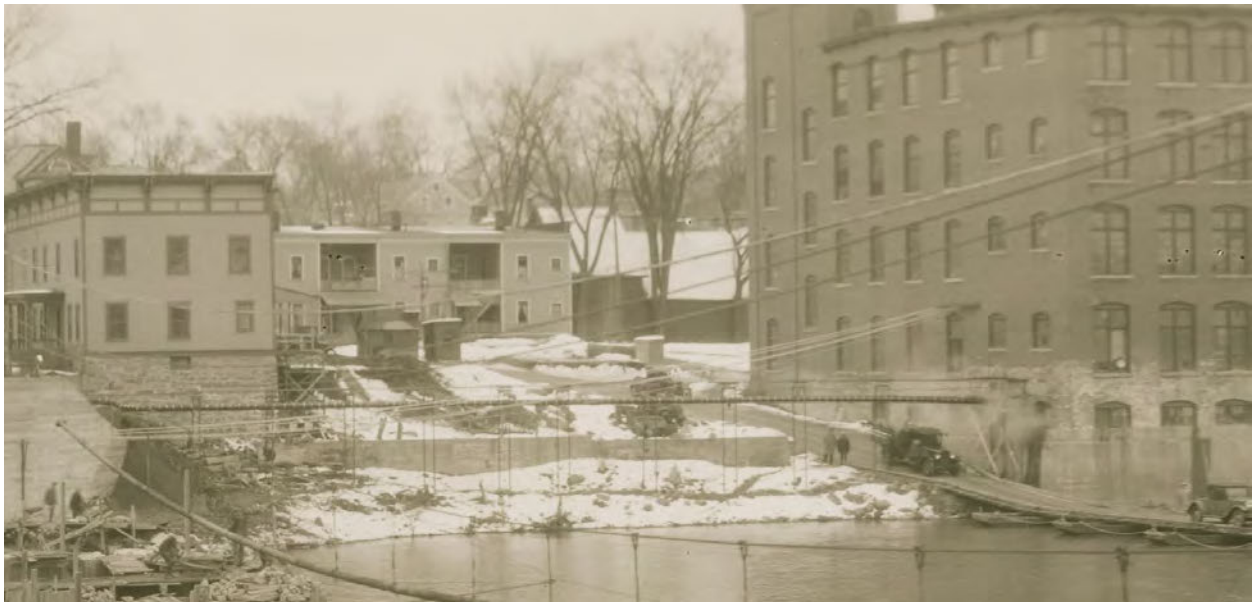
Figure 38. Detail of post-1927 flood photograph of the Winooski Bridge construction, showing the north end of the temporary pontoon bridge (Lois L. McAllister Photographs Collection, Box A19, Folder 13, Item 02, Silver Special Collections, Billings Library Annex, University of Vermont, Burlington, Vermont).
