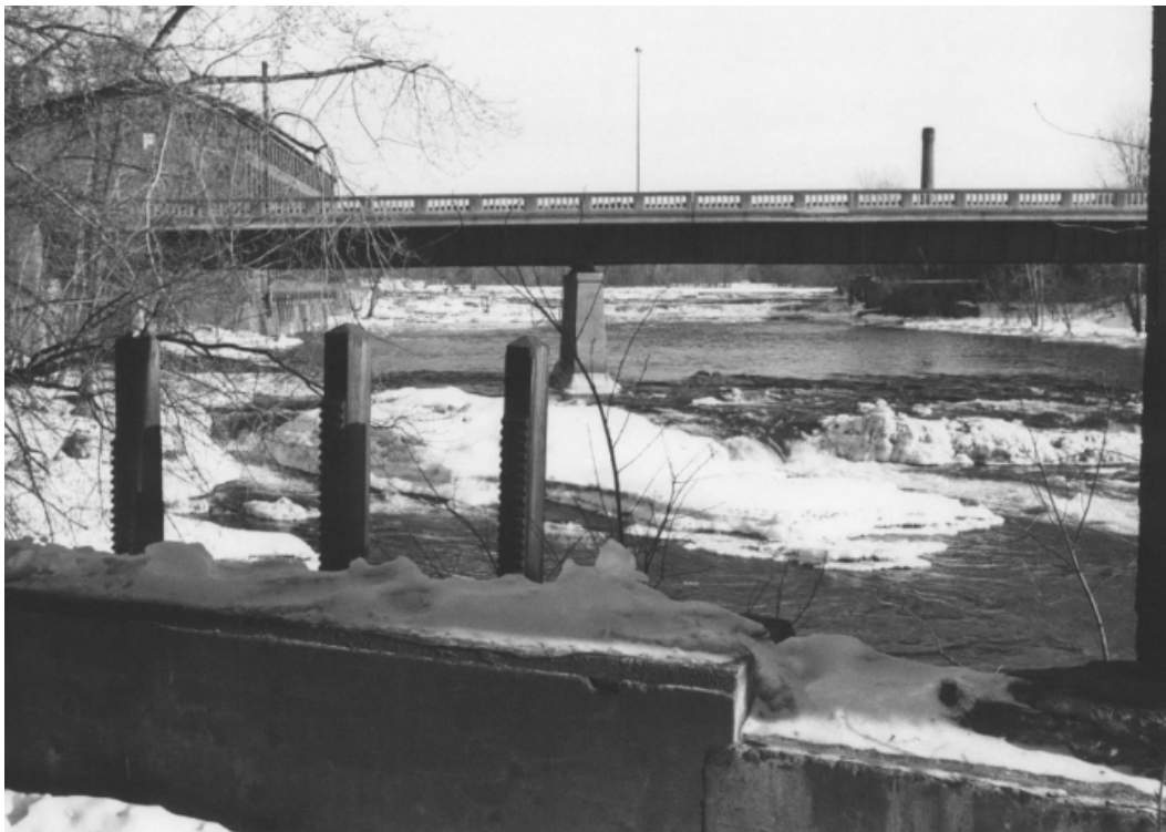
Figure 24. View looking up the Winooski from the Winooski Falls Mill District (National Register Documentation, Photograph #6; Credit: Hugh A. Boyd, April 1978). Note the gate stems (but not the gate hoist mechanisms) still in position.
