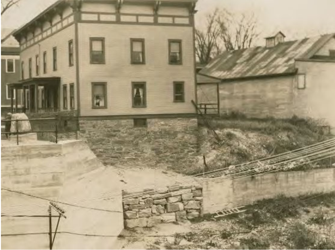
Figure 36. Detail of a view of Main Street Winooski ca. 1927, very shortly after the flood, showing the hotel livery / barn at right and the ca. 1898 three tenement building at left (Lois L. McAllister Photographs Collection, Box A19, Folder 07, Item 01, Silver Special Collections, Billings Library Annex, University of Vermont, Burlington, Vermont). The area to the right side of the livery / barn would be where pontoon approach would be located.
