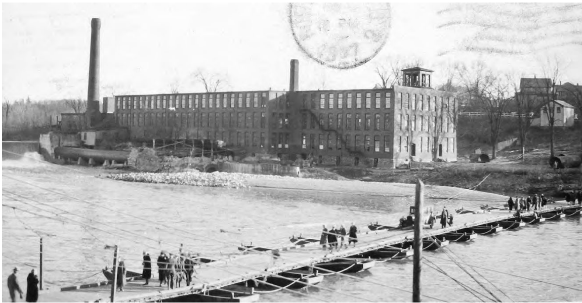
Figure 70. View of the temporary pontoon bridge crossing built after the Flood of 1927, looking southeast from the north bank of the river (Postcard Collection, Vermont Historical Society, Leahy Library, Barre, Vermont). Note wheelhouse and penstock at left (remains of which designated VT-CH-1300).
