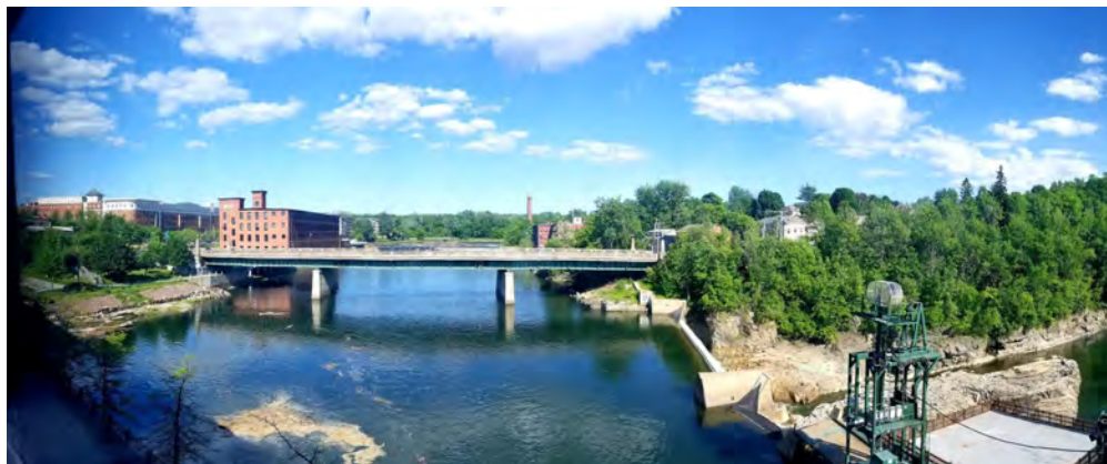
Fig. 1 - Existing Winooski River Bridge Looking East
