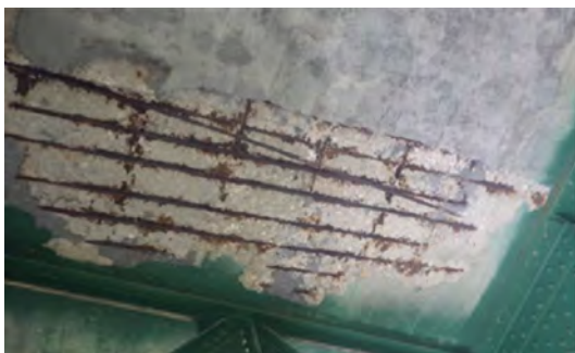
Fig. 4 - Typical Exposed Deck Reinforcing Under Deck
