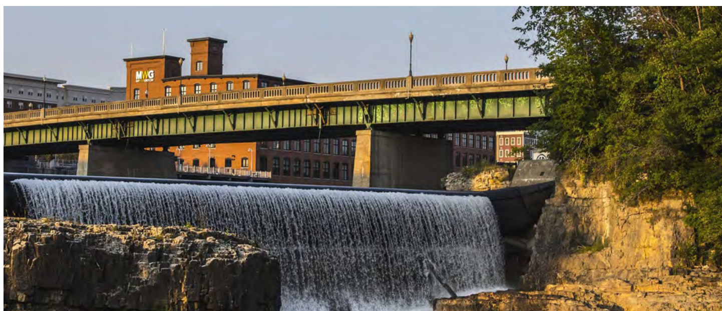
Fig. 13 – The Dam Located Just Downstream of The Bridge Provides Power to Both Cities
