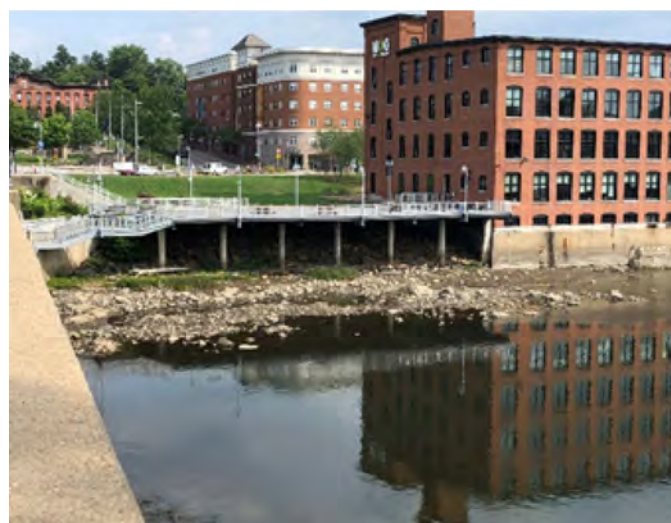
Fig. 11 – Looking North at the Riverwalk Deck and Mill Building
