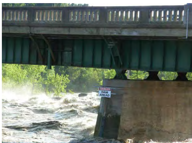
Fig. 18 - Eliminating a Pier Reduces the Vulnerability to Flood Events
