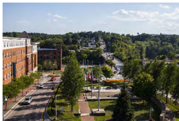
Fig. 7 – Looking South at the Winooski River Bridge with Rotary Park in the Foreground
